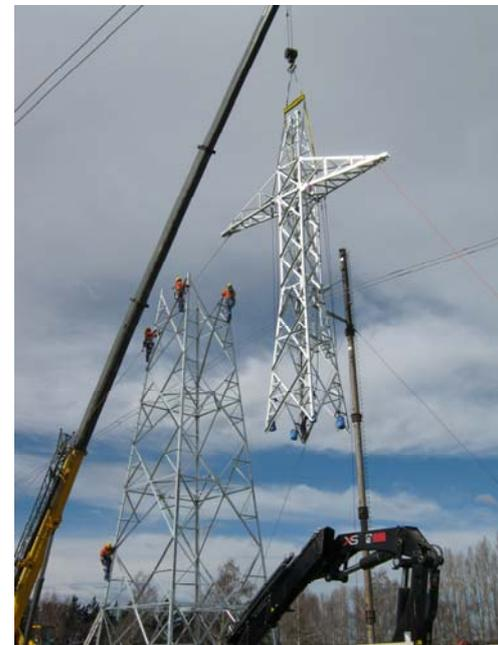
before conductors and earthwire could be reinstated. Redundant towers were disassembled for disposal by the separate tower assembly crew, and the sites reinstated.
